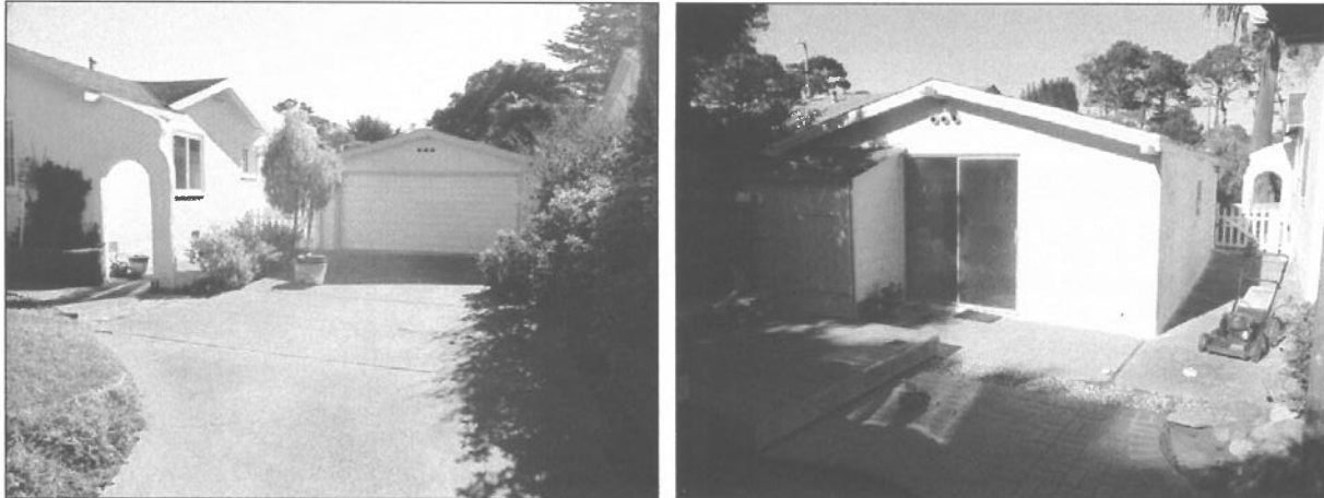
Figures 3 and 4. Left image shows the circa-1960s replaced garage to the right of the existing residence. Right image shows the garage's rear building wall with circa-1960s aluminum sliding doors installed in the rear-building wall.
