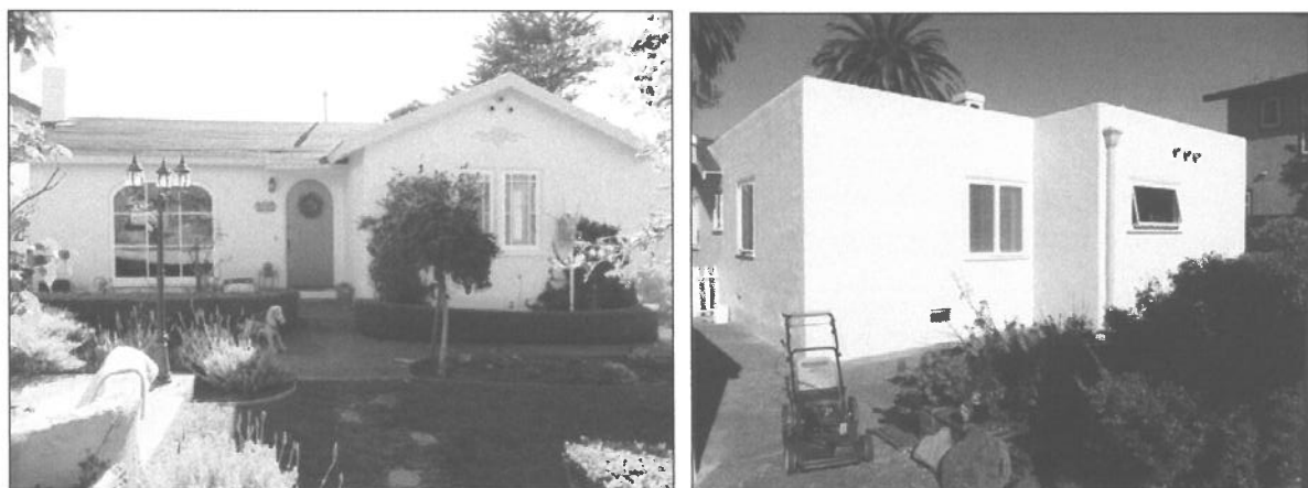
Figures 1 and 2. Left image shows the front elevation of the residence, with gable roofs, arched window and door openings and Spanish Eclectic-style decorative details. Right image shows the circa-1970s rear addition, with newer window technology in the openings.
